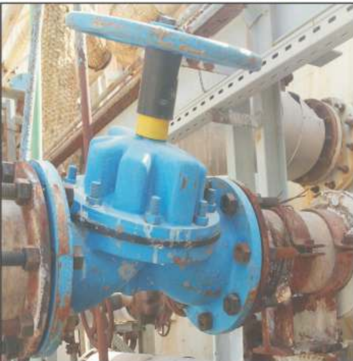
FEP Lined Diaphragm valve in Petrochemical Acid line
